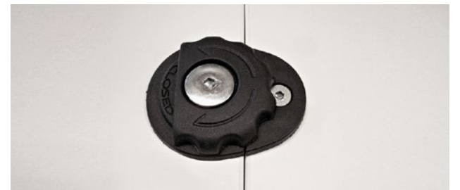
Anchoring by means of plastic clamp e=4mm
